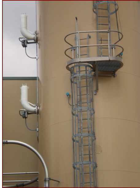
Fike HRD containers (vessel suppression)
