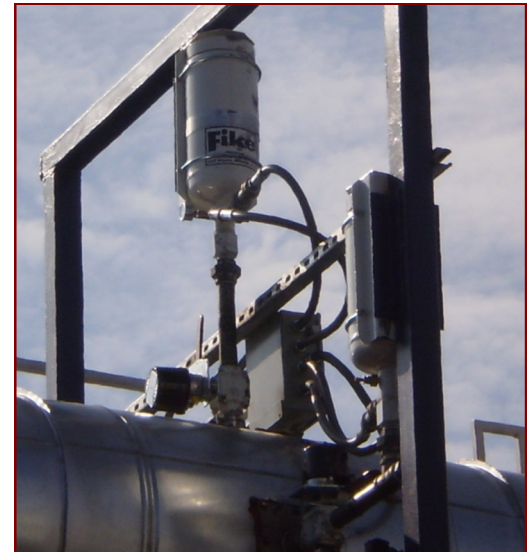
Fike SRD container (duct isolation)
